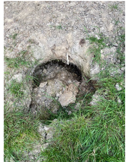
Figure 5: Entrance collapsed by cows
